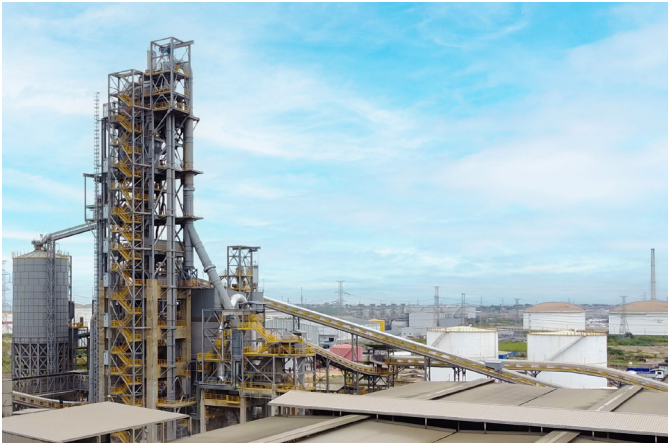
Above: Calcined clay plant in Tema, Ghana
