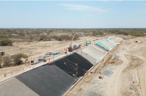
Cementos Pacasmayo in Peru has extended Cement Soil Stabilisation beyond pavements into riverbank defences to protect vulnerable communities from extreme weather events, saving 20% of CO 2 emissions. Read more on p46
