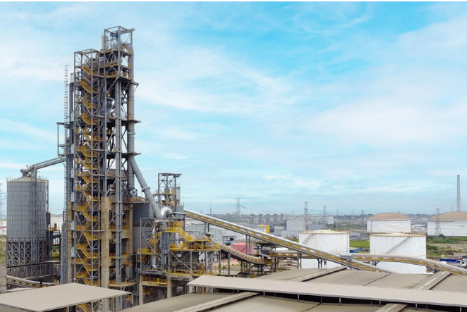
Above: Calcined clay plant in Tema, Ghana
