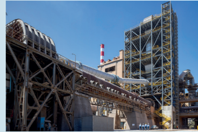
Above: Pre-calciner, Kamari cement plant, Greece
