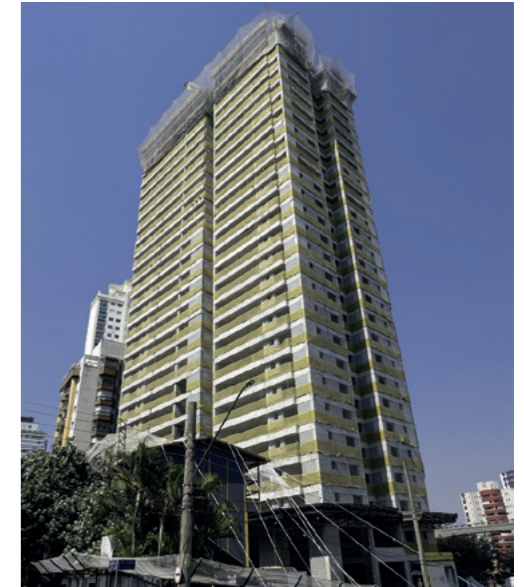
Votorantim Cimentos' Spectra product has been used by the project team on a 36-storey project in Brazil to optimise total concrete and steel use and reduce water and carbon emissions. Read more on p80.
