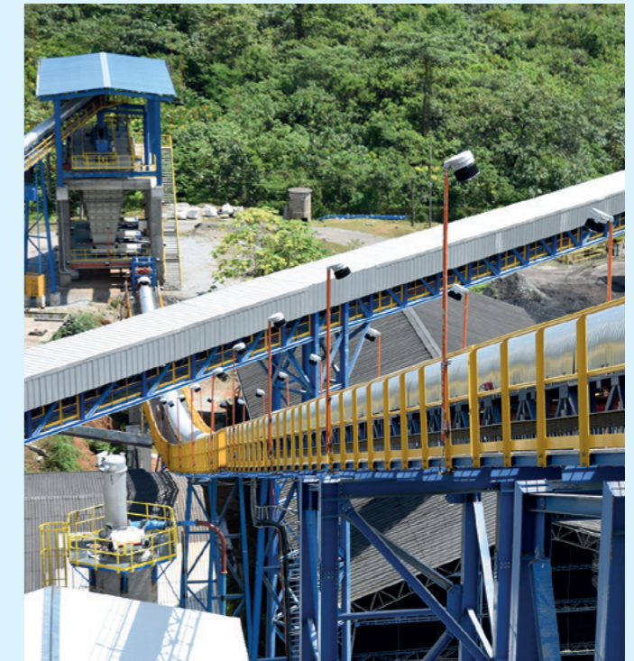
Above and above left: Rioclaro Plant, Colombia
