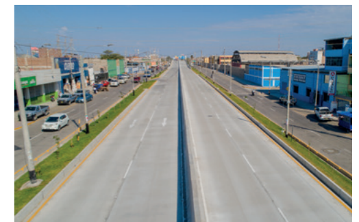
Only 14% of roads in Peru are paved, placing the country in the lowest quartile according to World Economic Forum. Cementos Pacasmayo promotes optimised slab concrete roads which deliver a 32% carbon reduction. Read more on p44.
