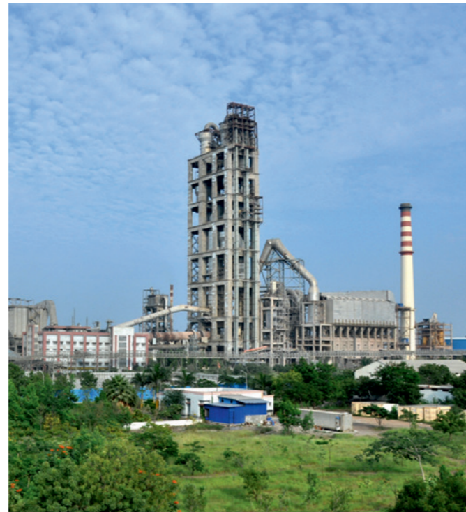
Above: JK Cement, Muddapur, India
