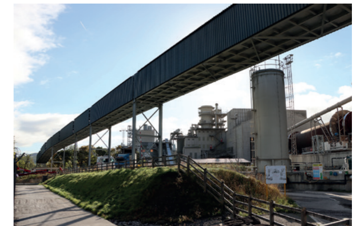
Top: Kinnegad Solar Farm Above: High-level conveyor installation for ARM at Hope Plant
