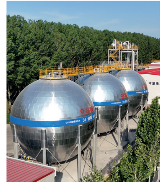
CNBM's CCUS project in Qingzhou Zhonglian, China commenced operation in January 2024 producing 200,000 t CO 2 /annum, exceeding 99.9% purity and an energy consumption 40% lower than alternative methods. Read more on p50.
