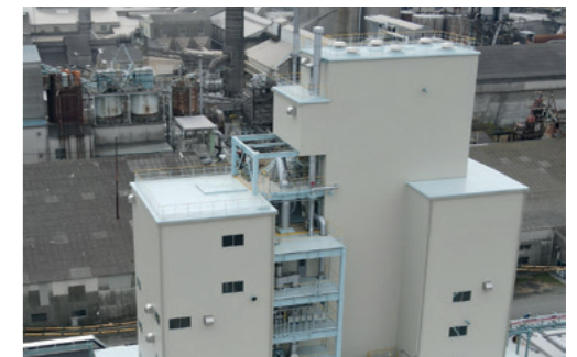
Taiheiyo is running carbon capture demonstration equipment installed in March 2024 in Japan . The compact facility replaces the conventional calciner. They are developing technology to convert recovered CO 2 into synthetic methane too. Read more on p71.
