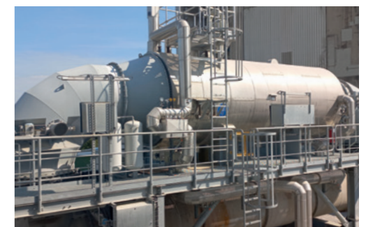
Buzzi has installed an innovative Organic Rankine Cycle (ORC) facility at its Geseke plant in Germany . This utilises previously unused waste heat to generate electricity equivalent to the consumption of around 250 four-person households. Read more on p36.
