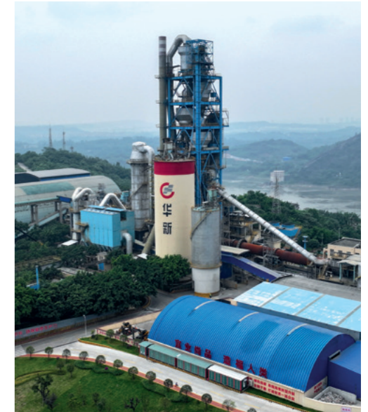
Huaxin has achieved a stable fuel substitution rate of more than 60% using alternative fuels such as waste tyres, waste rubber and waste textiles at its Diwei 2500t/d clinker line in China . Read more on p55.
