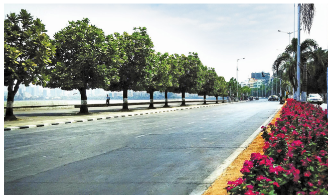
Figure 2b. Re-constructed as Concrete Road in 2012 after more than 70 Yrs.
