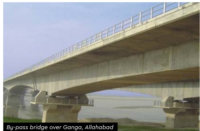
By-pass bridge over Ganga, Allahabad
